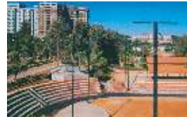
The mini-stadium and amphitheatre as seen from the terrace of the project office. Mayflower Block is seen at the far left and Magnolia Block next to it.
