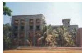
The school building nearing completion, as seen from the mini-stadium.
