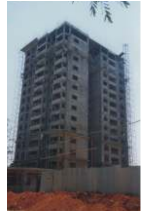
Magnolia Block construction nearing completion.
